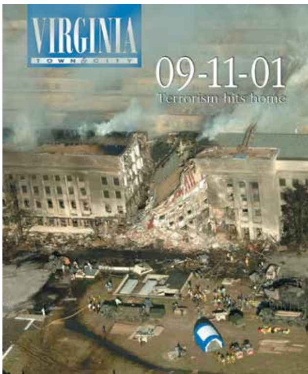
2001: Sometimes a picture is all that's really needed. Interesting fact: This photo of the Pentagon after the September 11 attacks was taken by Scott Boatright of the Fairfax County Fire and Rescue who sent it directly to VML's Manuel Timbreza. It appeared on the cover of VTC first.
