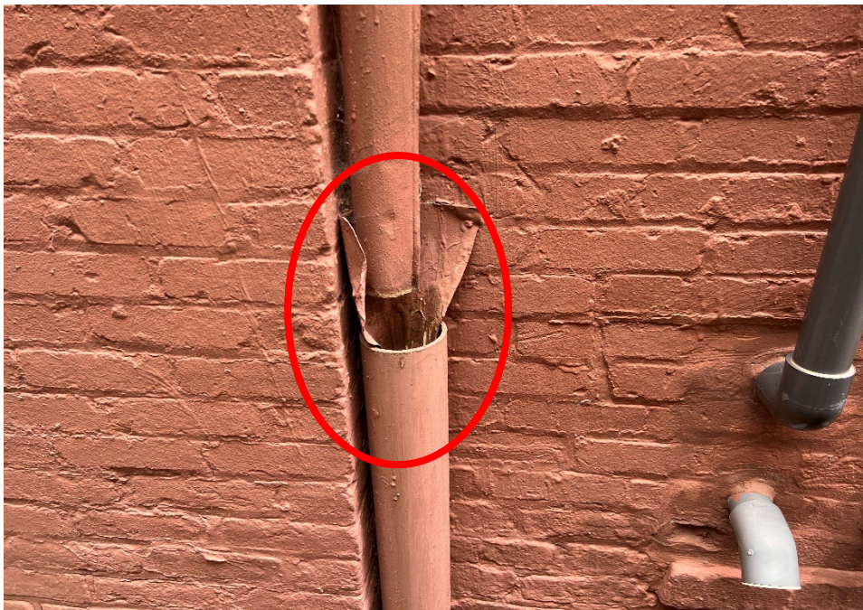
Several of the gutter downspouts discharge into the city's stormwater system.
